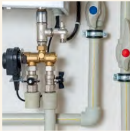
+ 24 Hrs Water Supply
